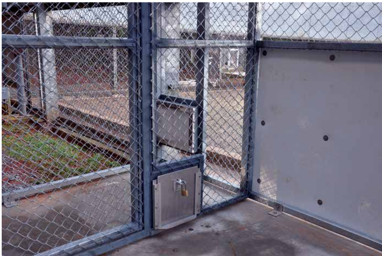
Figure 2. Capture unit inside the introduction enclosure. The capture unit is a 1.16 m × 2.87 m enclosed space behind the enclosure proper. The locked sliding door here separates the 2 areas.
