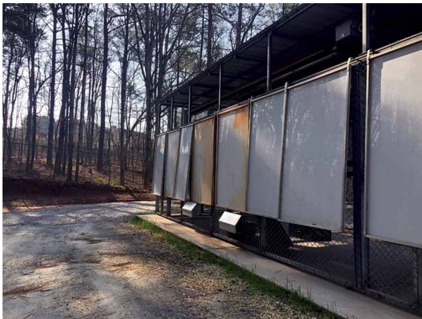
Figure 4. Enclosure with infrared gas tube heaters and hanging polypropylene panels.
