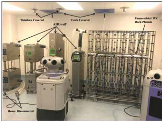
Figure 4. Static–open VHP exposure, with ceiling thimble connections and HVAC supply and exhaust vents covered, all AHU off, hoses left disconnected, and the IVC rack left unassembled and unconnected to an AHU.
