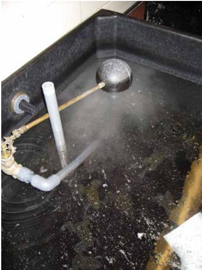
Figure 2. Milky-white, turbid water with visible gas bubbles entering the X. laevis pond-style holding tank. As described in the case history, this water was supersaturated with entrained air (total dissolved gas concentration exceeded 112%; less than 100% is normal).
